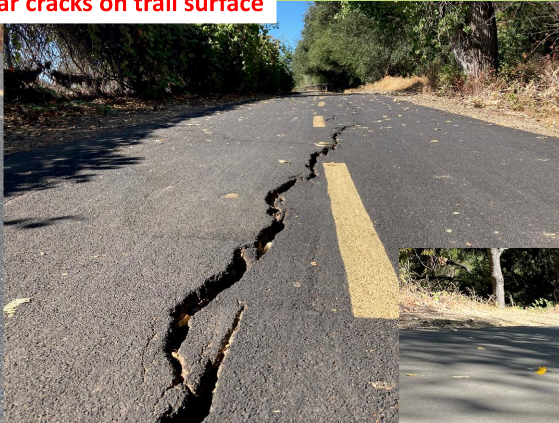
Linear cracks on trail surface
